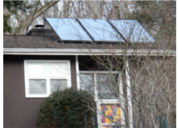
Solar Domestic Hot Water collectors
