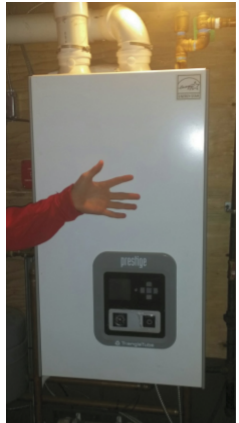
High-efficiency condensing gas boiler. Hand shown for relative size.
