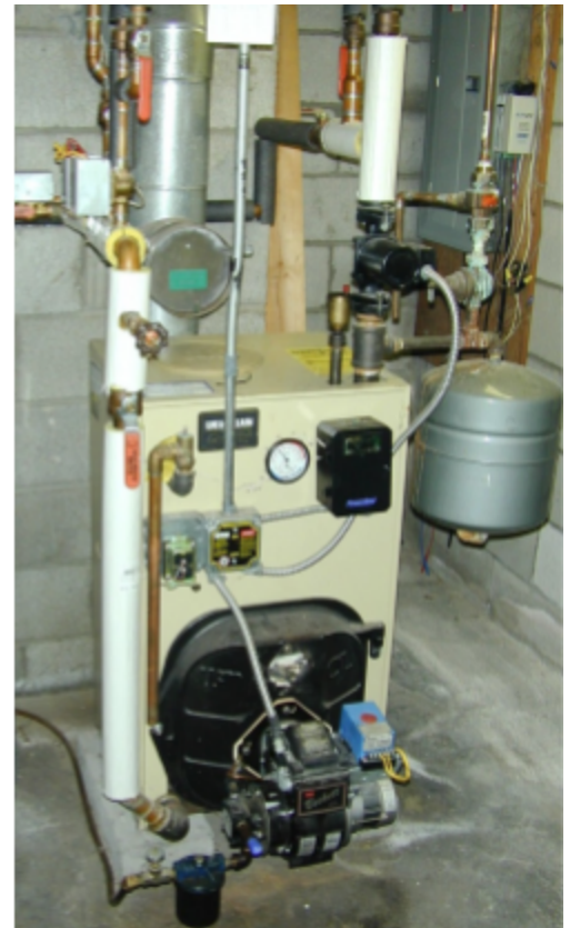
Typical oil-fired hot water boiler
