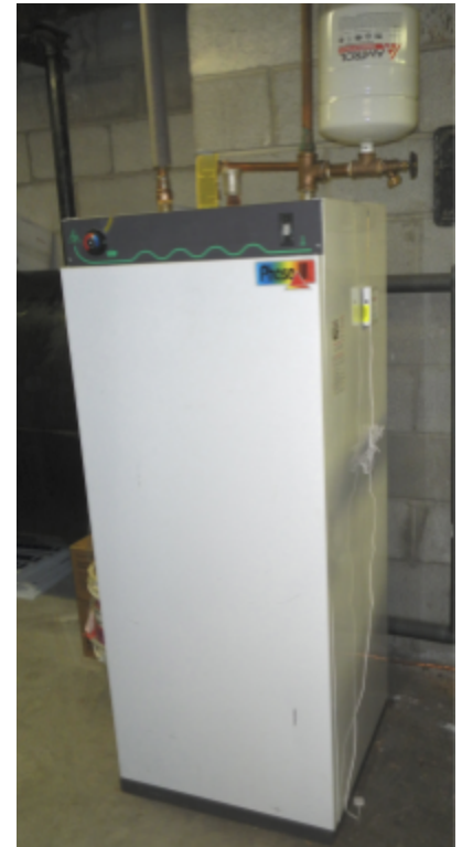
Indirect DHW heater piped to a boiler
