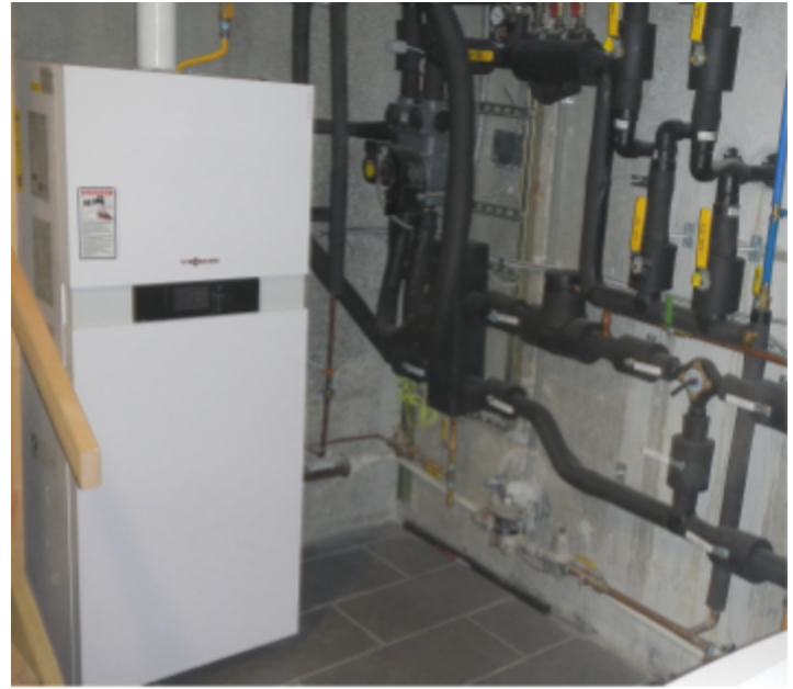
Ground source heat pump and piping
