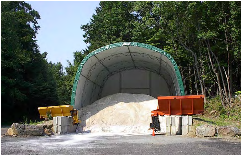
Current Salt Storage Facility for the Town of Ossining, NY
