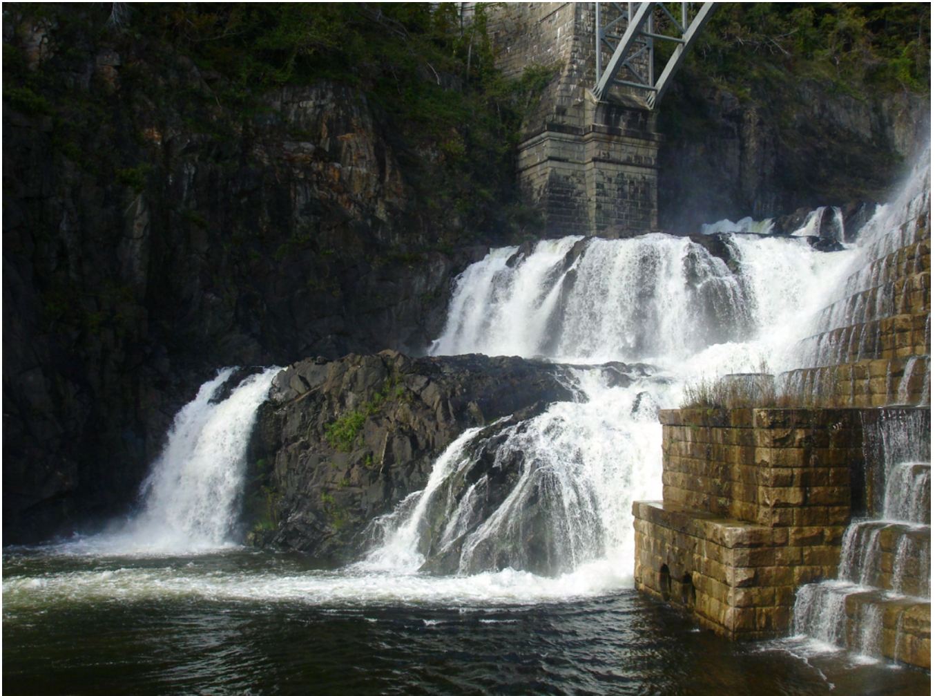
Figure 2-29. Croton Dam Falls, Cortlandt, New York
