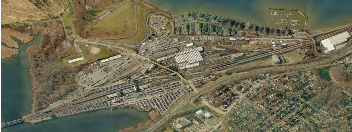
Croton-Harmon Metro-North Railroad Station and Harmon Yards (Source: Bing Maps)
