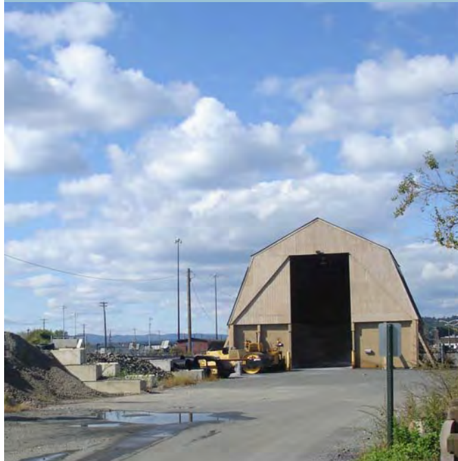
Figure 2-27. Municipal Garage, Croton
