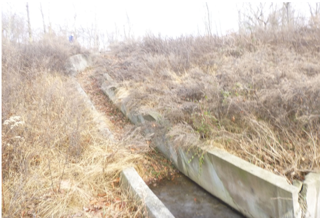
Photo 5 Dam ID# 214-5260 Hudson National Golf Course Detention Pond Dam 01/06/2022 Spillway chute
