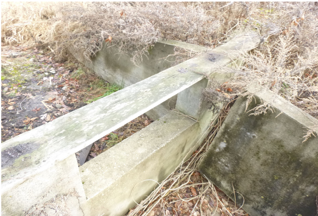
Photo 4 Dam ID# 214-5260 Hudson National Golf Course Detention Pond Dam 01/06/2022 Spillway inlet looking upstream
