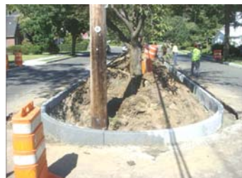
Curbing being installed
