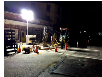
Nighttime valve replacement at dummy light on Grand and OPRS
