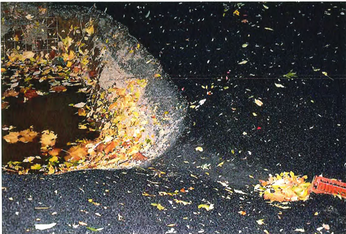
2016: the trench flows to an ad hoc open sediment collection ditch, which now receives all of the water from the expanded maintenance yard and the water from the lower golf course part of Prickly Pear Hill Road.
