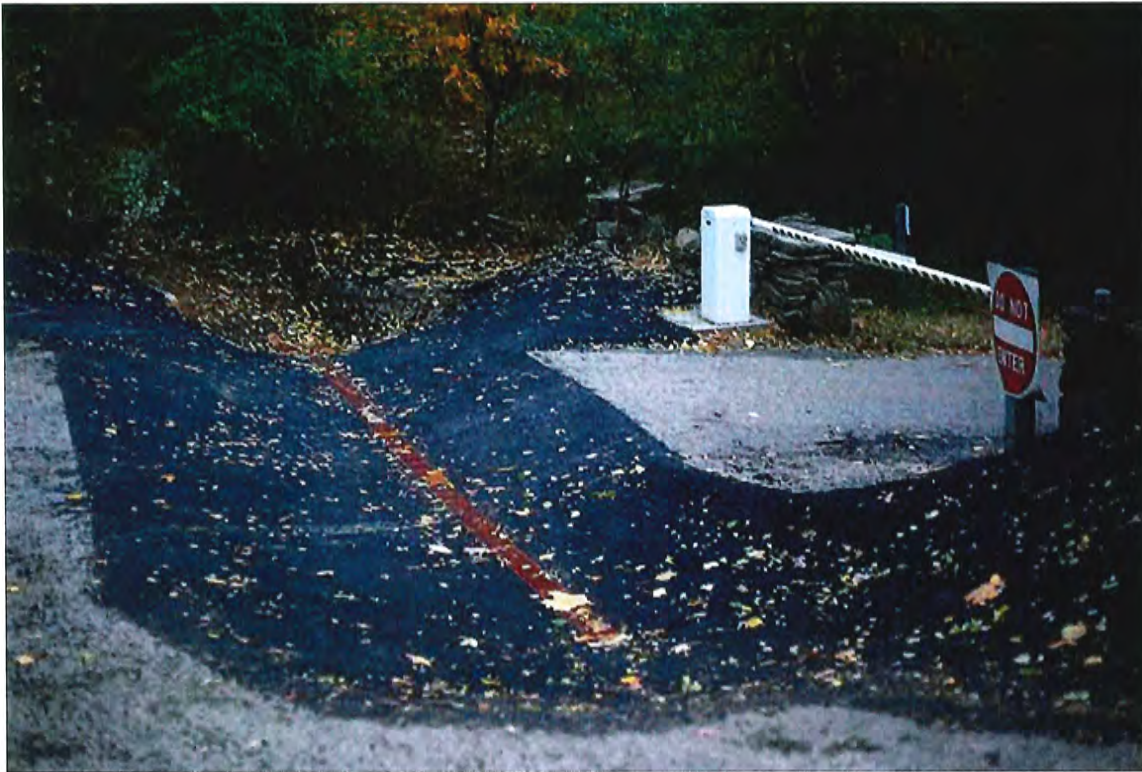
Trench installed in Fall 2016. It would have prevented emergency vehicles from gaining access to the golf club.
