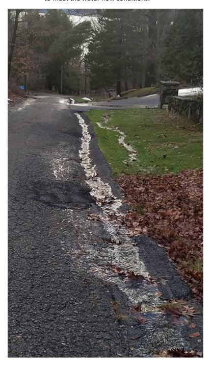
D. We saw two culverts at the end of Prickly Pear Hill. One conducted water from the north swale of Prickly Pear Hill Road to the South and on to the 9A western swale. The other culvert transverses Prickly Pear Hill Road connecting the swales along the 9A hiway. Both culverts will overflow onto both roads during a significant rain. Much can be improved if the culverts were properly maintained and cleared of debris on a regular basis.
